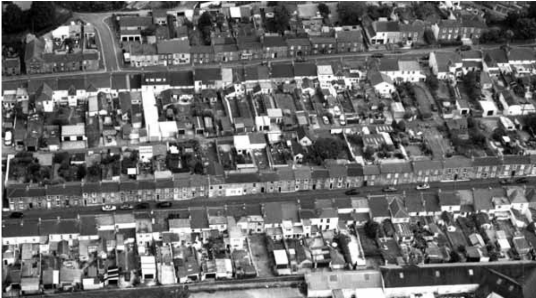
Tuckingmill, Camborne. The town of Camborne and the Camborne/Redruth conurbation contains the best example in Cornwall of large-scale urbanisation associated with the Industrial Revolution. The townscape is dominated by industrial terraces, many of which remain largely unaltered. Photo © Cornwall County Council Historic Environment Service
