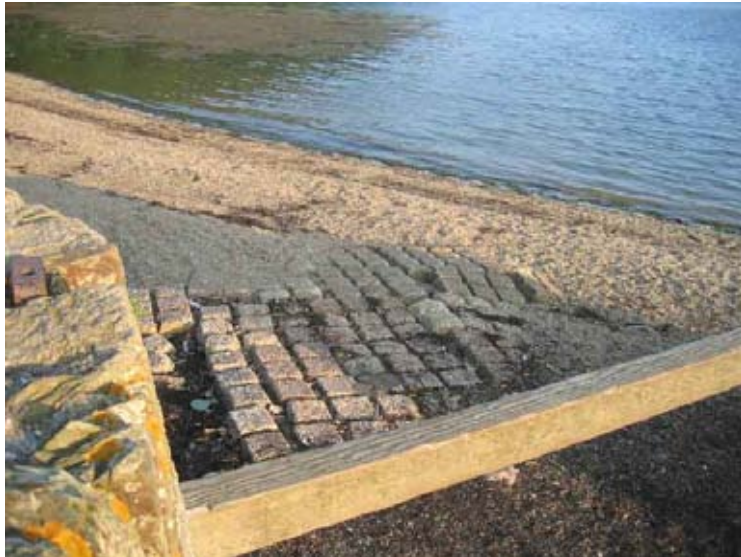
Remains of some of the flexible concrete matting from the D Day hard at Turnaware. Photo © Cornwall County Council Historic Environment Service
