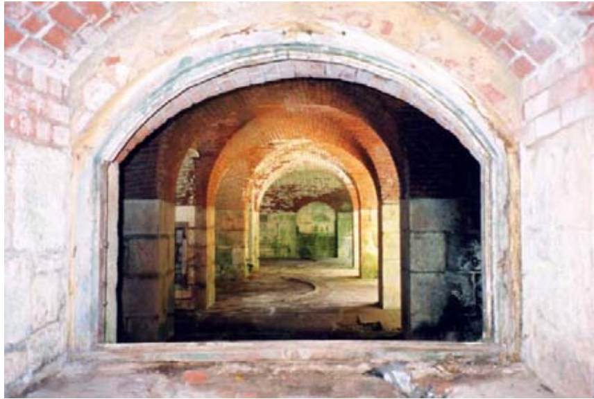
The interior of a gun casemate at Scraesdon fort. Photo: Emma Trevarthen.
