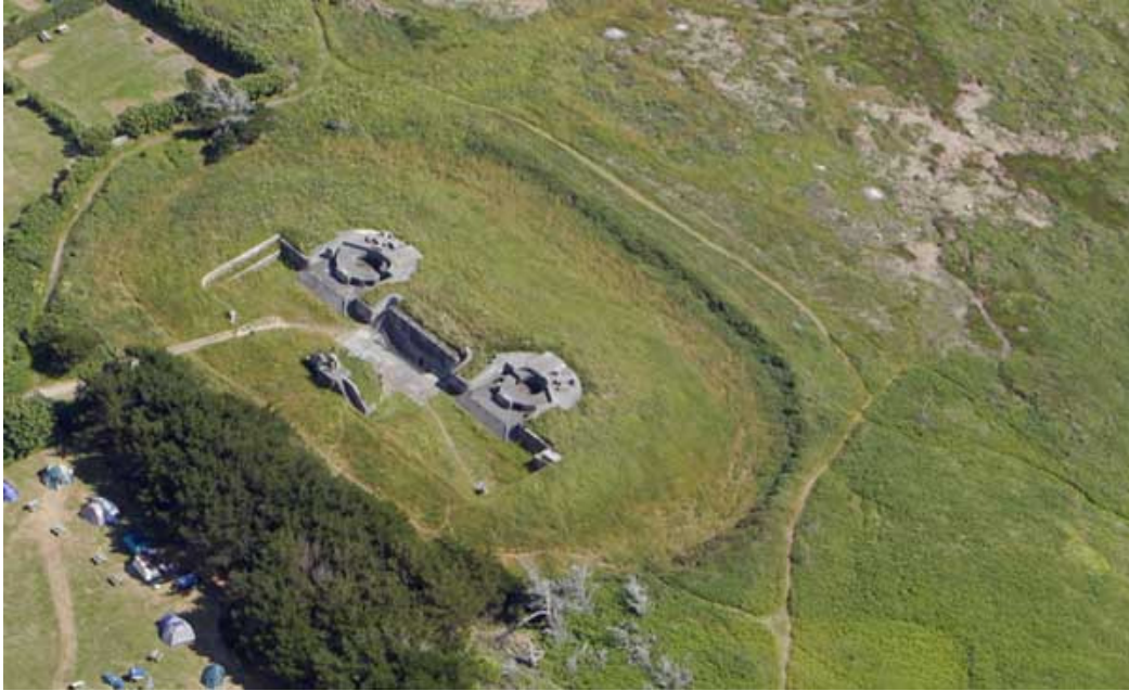
A gun emplacement at Woolpack Battery, the Garrison, St Mary's. Woolpack is a well-preserved 1900s fort, commanding the southern shoulder of the garrison headland, with its pair of Defence Electric Lights on the clifftop below. Within the rampart of the battery are gun emplacements above sunken shell and cartridge stores and shelter rooms. Photo © Cornwall County Council Historic Environment Service
