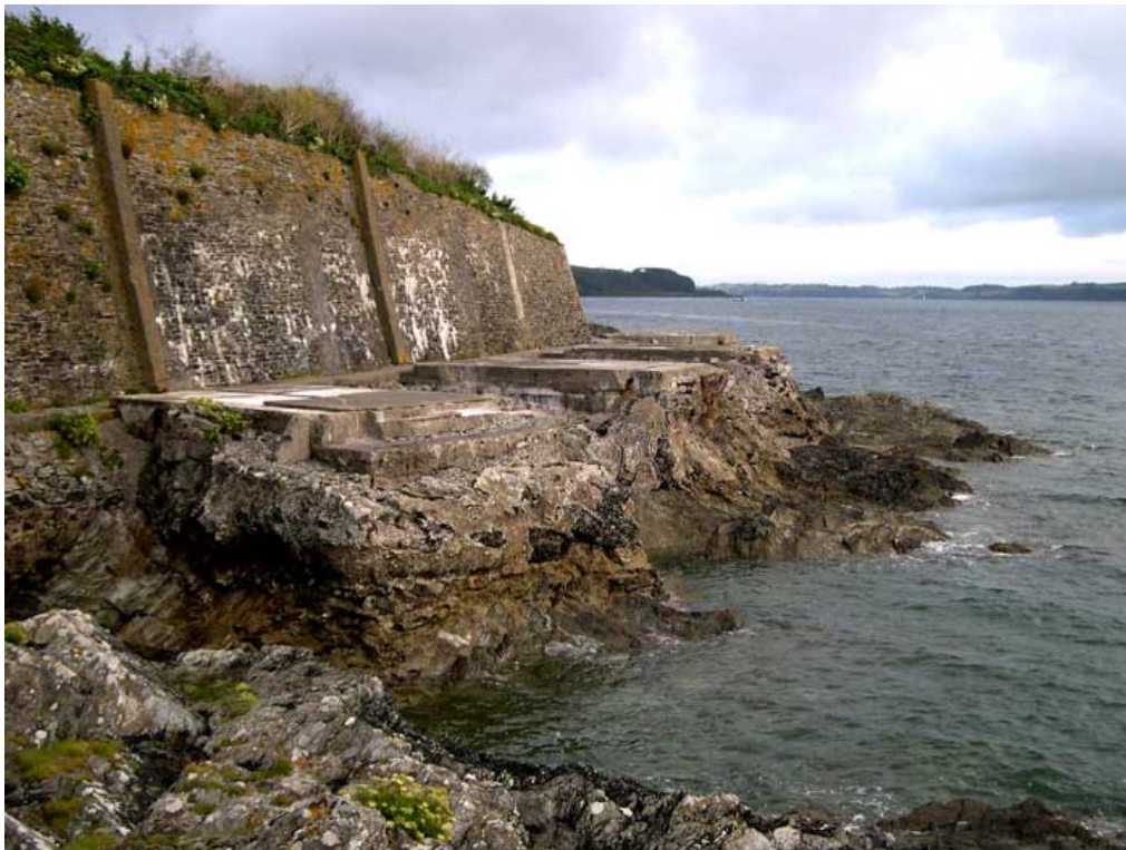
The remains of bases for Defence Electric Lights at Crab Quay on the edge of Pendennis Headland. © details
