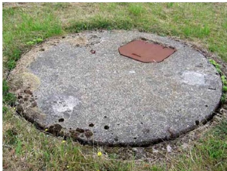
One of the Pickett-Hamilton forts at RAF Cleave showing how the concrete lid fits flush with the ground.
