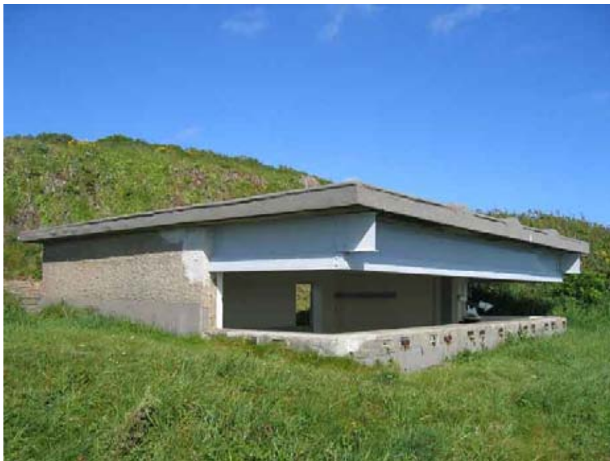
An observation post at St Anthony Head battery. The gun emplacements and other operational buildings of Second World War coastal batteries were protected against aerial attack by reinforced steel and concrete roofs. Photo © Cornwall County Council Historic Environment Service
