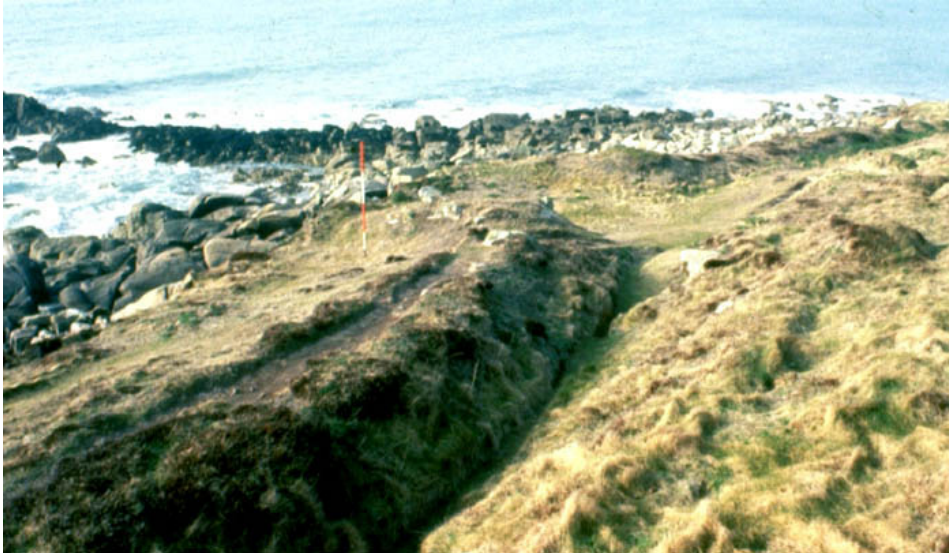
Part of the breastwork on the Garrison, St Mary's. The earthwork bank, which was stone-faced, is accompanied by an inner ditch. Towards the centre right of the photo is a protruding battery. This cliff-top defence is a remarkable survival from the English Civil War. Photo © Cornwall County Council Historic Environment Service
