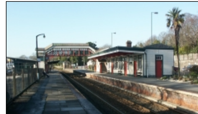
The integrated rail and bus station is potentially a major asset as a visitor 'gateway'
