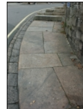
Distinctive high-quality surfacing enhances the character of the area
