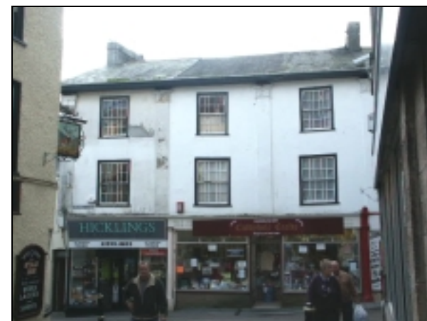
Nos 6-12 Vicarage Hill – a potential exemplar for a sensitive repair scheme
