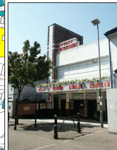
The Regal cinema, 1935, quality architectural contribution of its time
