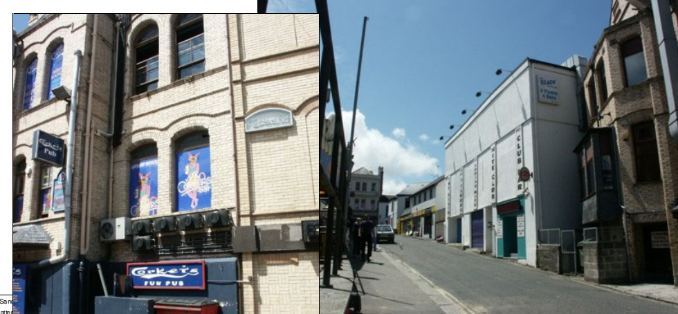
Enhance Beach Road and Gover Lane - screen service areas and activate street frontages. Strengthen links between the commercial core and the coastline
