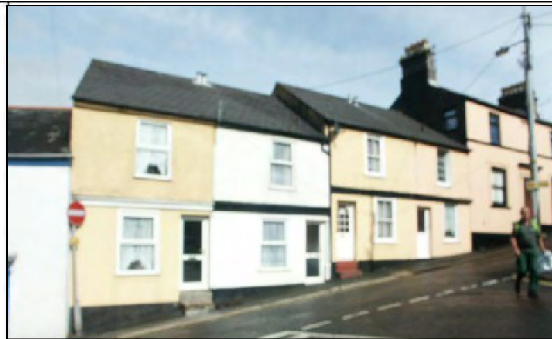
Although still retaining their essential character some of the historic integrity of these cottages has been lost through the use of modern replacement windows and doors
