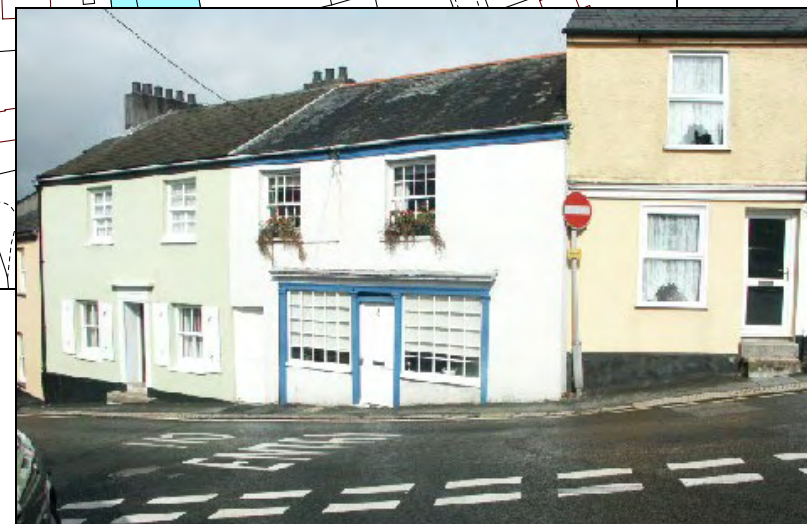
Former shop now converted to domestic use in Church Street
