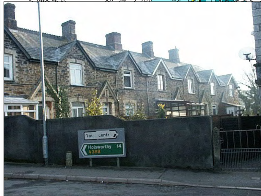
Windsor Cottages, Newport.
