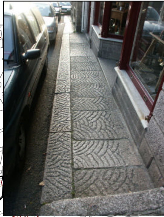
Narrow pavement and distinctive fan-scored granite surfacing at the south-west end of Wendron Street.
