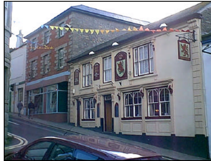
Buildings on the west side of Market Place. Diverse architectural forms and materials and the sloping topography contribute to the character of the area.
