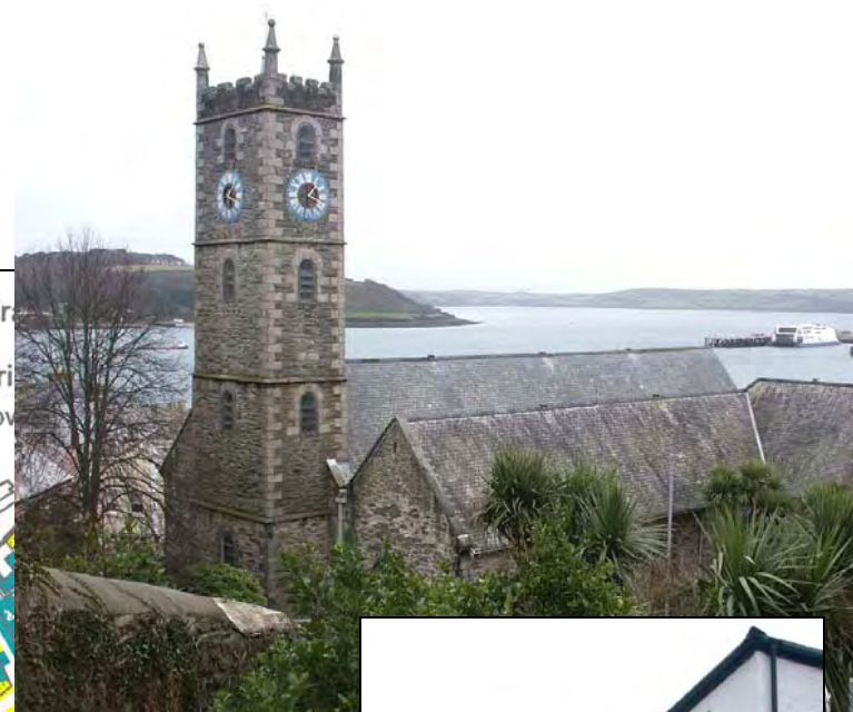
Falmouth parish church and views to Carrick Roads
