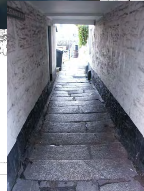
Open and paving, North Quay
