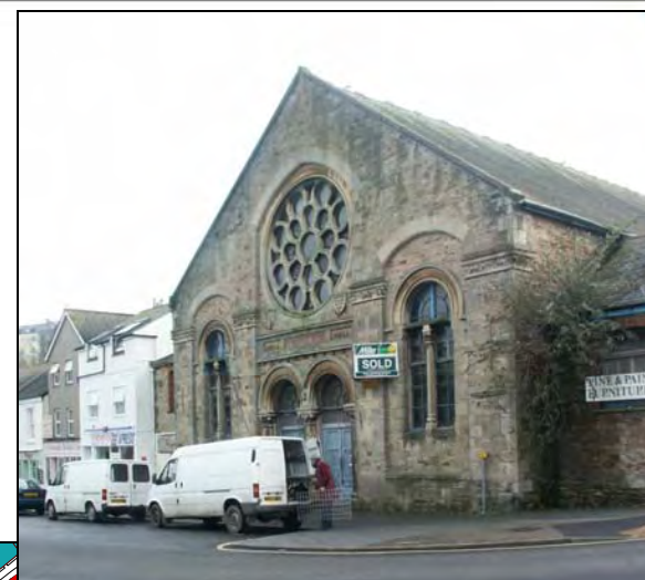
The Drill Hall
