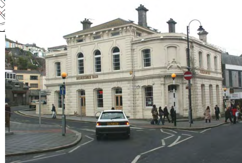
The former Town Hall
