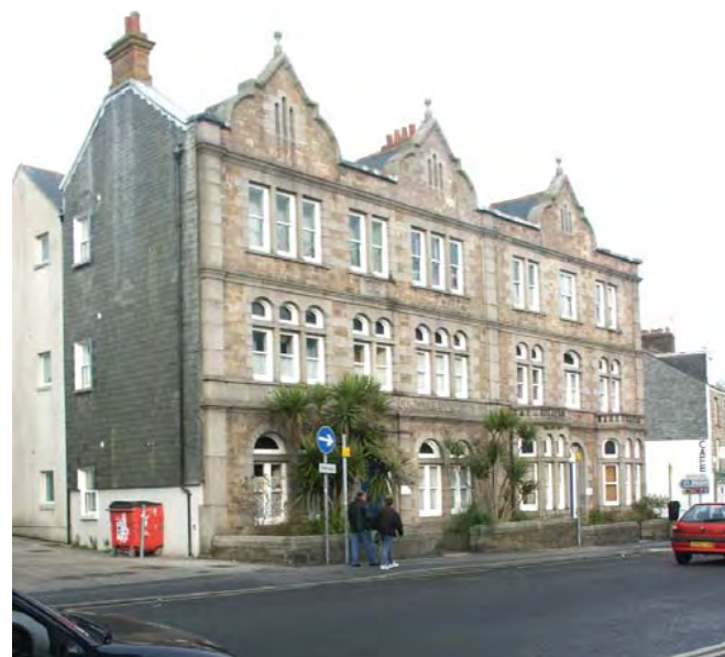
The former police station
