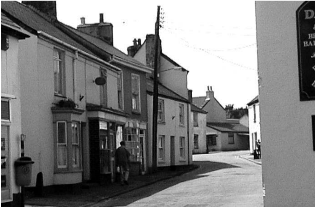
Figure 5 Fore Street looking west into the site of the medieval market place; early-mid 19 th century commercial buildings (left) [75] stand next to houses potentially much older [[74][72][100].
