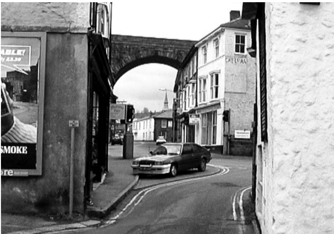
Figure 6 Penryn Street from Cross Street, the core of the medieval settlement, looking south to 18 th century expansion [347] and high class redevelopment [267-280] associated with the building of the first viaduct in 1850-52, rebuilt 1884-8 [271]
