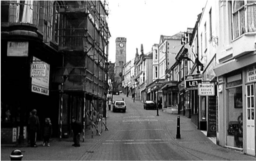
Figure 5 Fore Street looking east to the Town Clock [296], built 1828, heightened 1904, symbol of Redruth's commercial strength, the greatest market of west Cornwall from the 17 th to early 20 th centuries.
