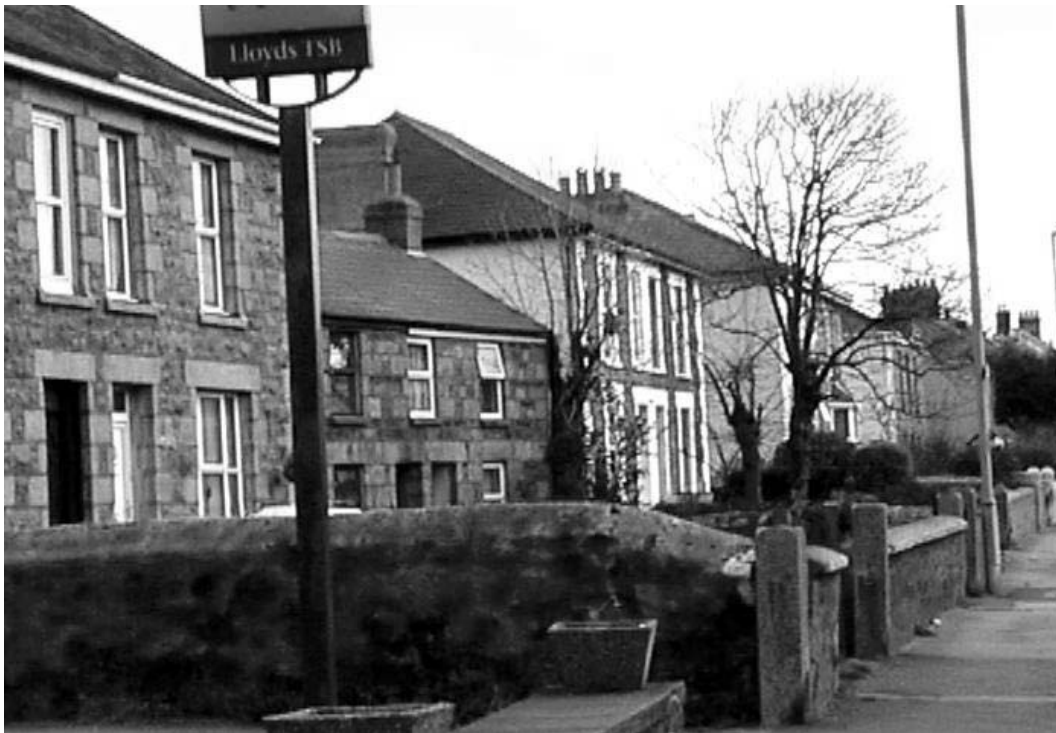
Figure 7 On the main street, smaller houses [6] set at an angle to the main road show the impact the new (1839) turnpike had on an older settlement pattern
