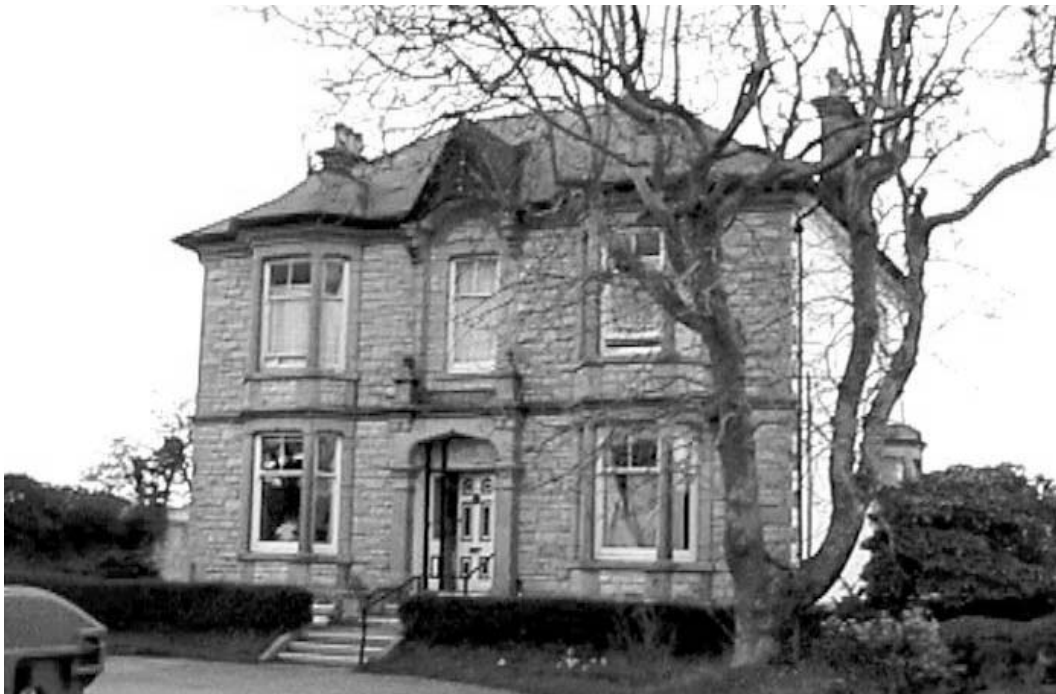
Figure 8 Teague House – the profits to be made from mining. Along and just off the main road are several quality buildings - School [84], Chapels [29-31], Almshouses [44], and this fine mine managers house [56].
