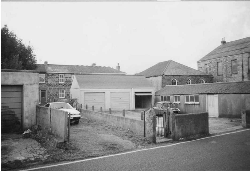
Figure 9 The quality of some very important historic buildings and streetscapes has not always been recognised in the past nor treated as sympathetically as it might have been (North Parade [222] [223][83]).
