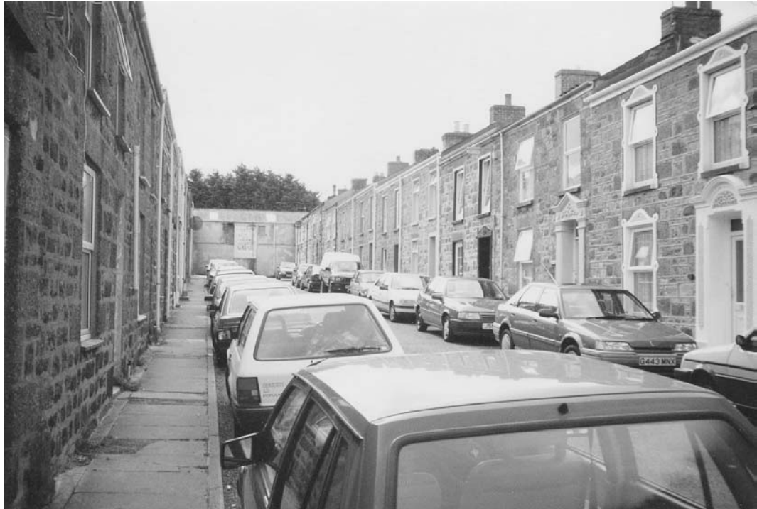
Figure 5 The overriding impression of Camborne – an industrial town with rows of workers' cottages, hard landscapes and tight urban grain, often in direct contact with relict industrial sites (East Charles Street [293]). Highly individual detailing lightens the street scene.
